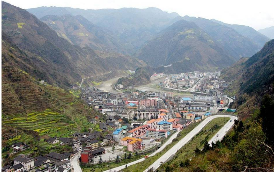
(Beichuan County before the Earthquake)
