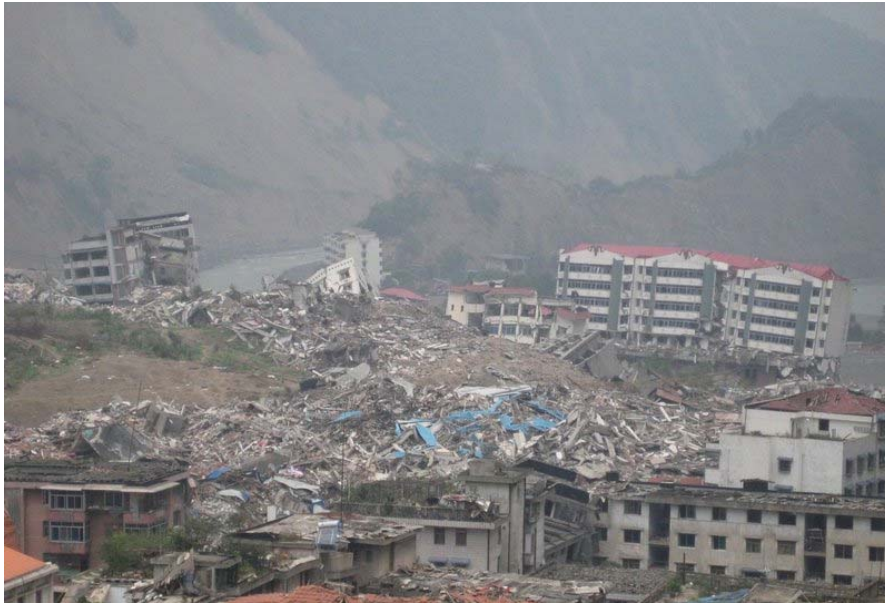
(Beichuan County after the Earthquake)
